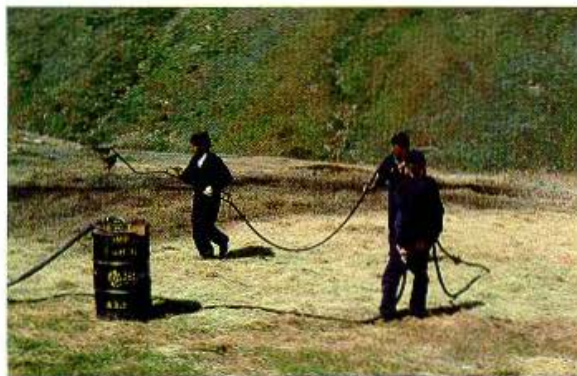
The old track between Carruthers Peak and Mt. Twynam was so deeply eroded it had to be filled with hay bales and covered with top soil before seeding, fertilising and bitumen spraying could begin. The final photo taken in March, 1985, shows the revegetated track with greater concentrations of snow grass alongside the fertilised areas.
