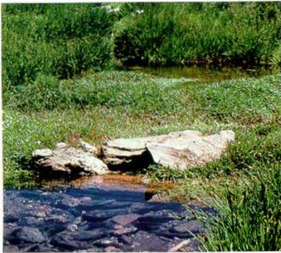
Stone weirs are built across creeks to reduce the velocity of water and trap sediment. Montia, a mat-forming creeping plant is transplanted by hand and slowly recolonises, once more bridging the creek.
