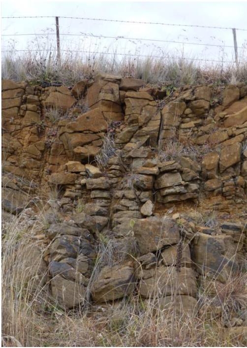
Figure 9. Basalt rock columns on Maffra Road, at Ravensworth TSR.
